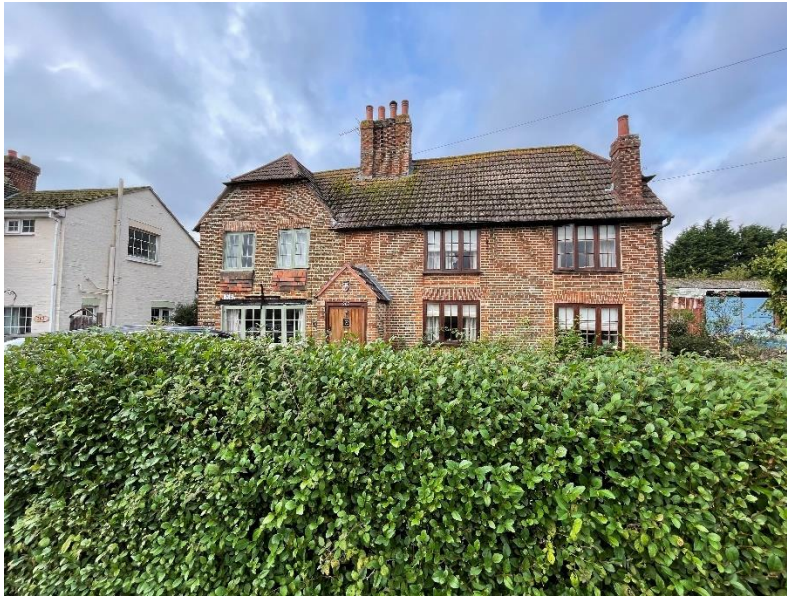
Plate 13: The Grade II Listed Foxbury Cottages, Foxbury Farmhouse, view west from Newbury Lane
